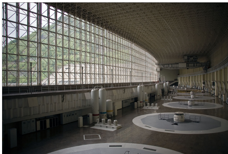
Figure 2.27: Sayano Shushenskaya's turbine hall before the accident where turbine 2 (the turbine that failed) is in the foreground of the image a .
