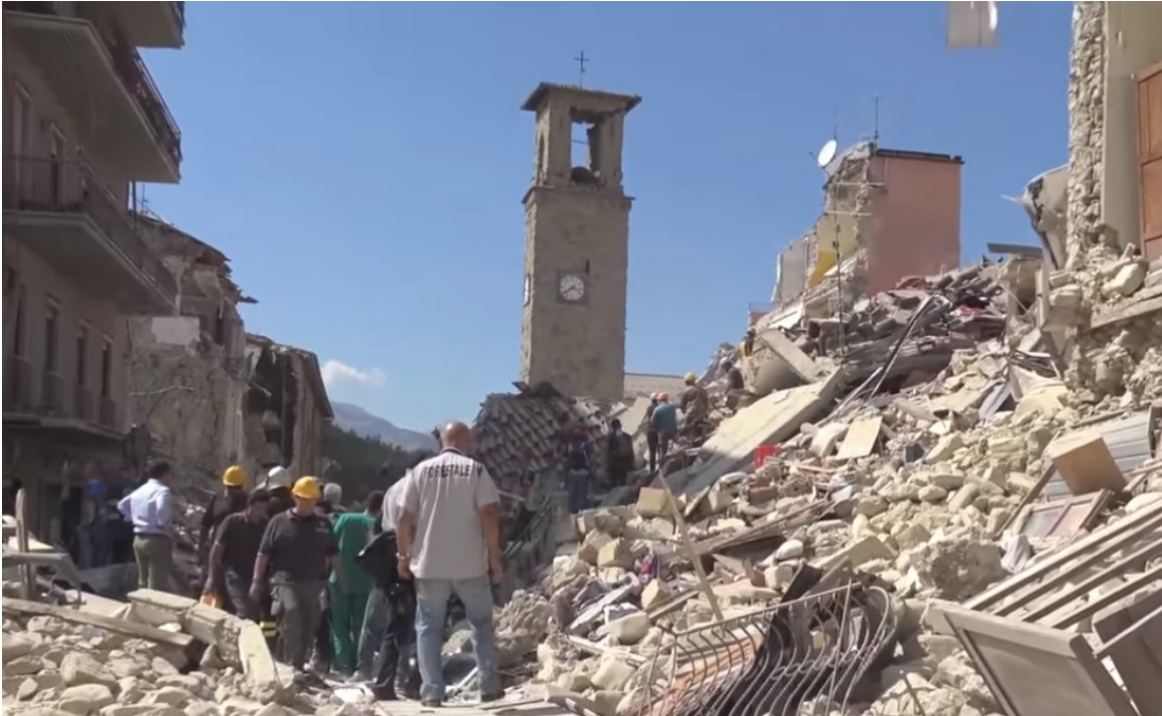
Figure 3.21: The town center of Amatrice Italy after the August 24 th 2016 earthquake that measured 6.2 on the moment magnitude scale; note that the bell tower (lower natural frequency) is still standing while shorter stiffer structures (higher natural frequency) have suffered extensive damage. a
