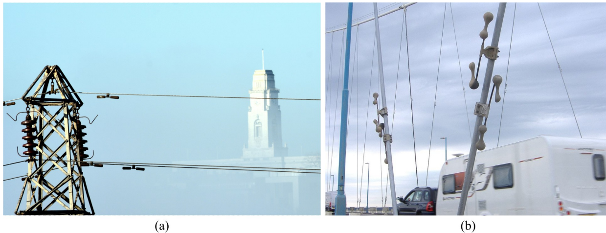
Figure 6.3: Vibration absorbers deployed on wind excited cables showing: (a) a Stockbridge damper on a high-power transmission line a , and; (b) a dogbone damper on a suspender cable of a suspension bridge b .
